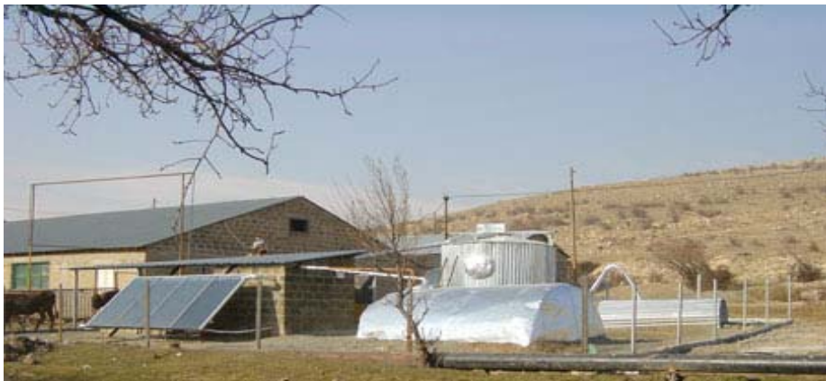
Bio gas plant in Lousagerd farm
